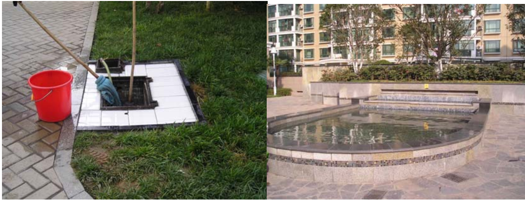
Figure 4-29: Reuse storm water for streets cleaning and for scenery in Nanjing Wanfuyuan Community
