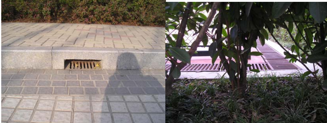
Figure 4-25: The storm water collection equipments for street in Nanjing Wanfuyuan Community
