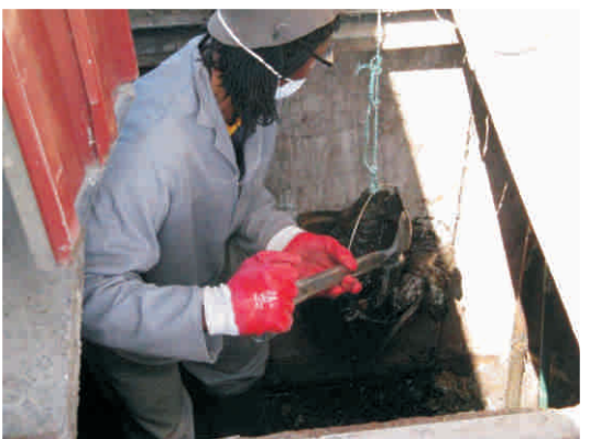
Figure 23 : Manual emptying of chambers
