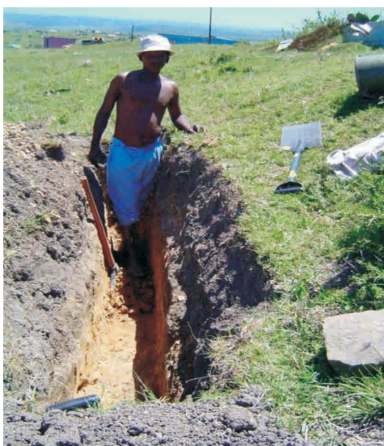
Figure 24 : On-site deep burial of sludge
