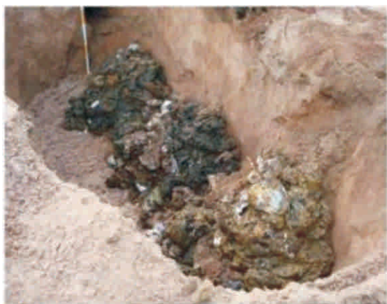
Figure 41 : Deep row entrenchment of pit sludges
