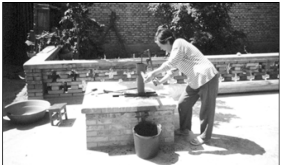
A typical water tank for household drinking water supply
