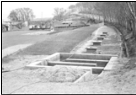
The paved highway is used for a runoff catchment
