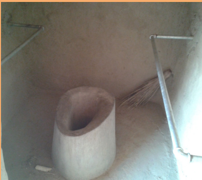
Fixed toilet seat with handrails. Rails could be made from wood to reduce cost. Credit: WaterAid/Jane Wilbur.
