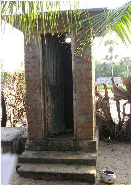
Toilet with high steps and narrow door, Batticaloa, Sri Lanka. Credit: WEDC/Hazel Jones
