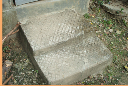
Low steps, cross hatched to make them less slippery when wet, Nepal. Credit: Jones et al 2009.
