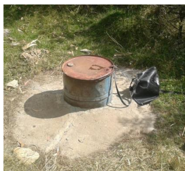
Photo 8: Simple well protection, Farta, Amhara; with bucket made of an old car inner tube lying by the well
