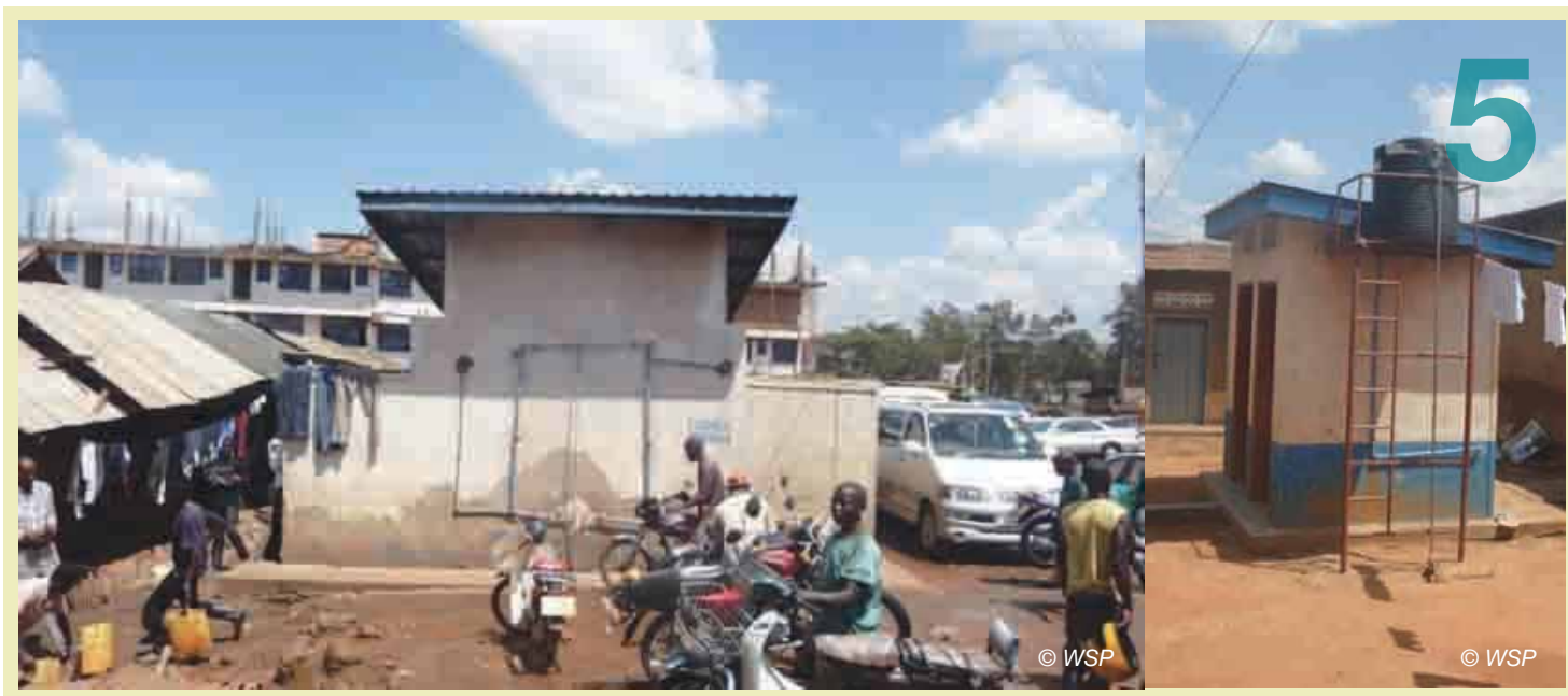
5 Picture 5: Public and private Sulabh toilets in Kisenyi (Kampala, 2011)
