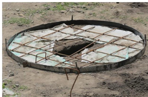
Figure 1 Iron bars laid for concrete slab production
