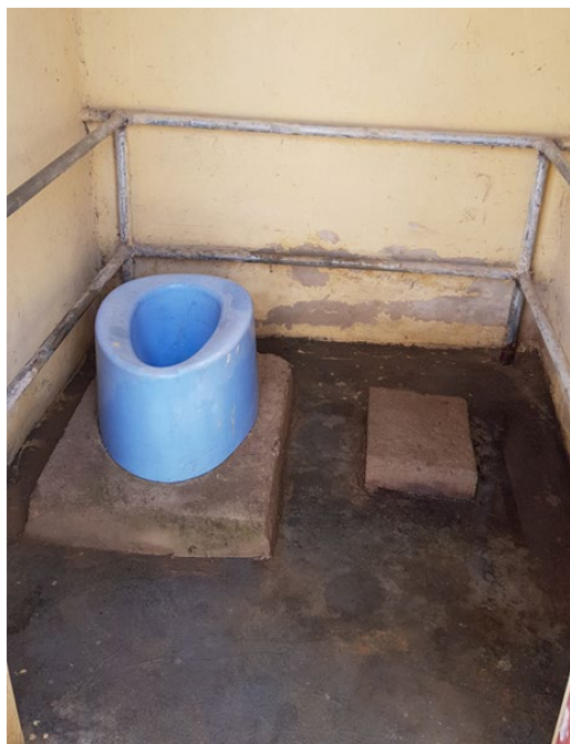
Figure 3: Sato stool constructed by a toilet business owner over a drop-hole latrine in a health care facility in Jigawa state
