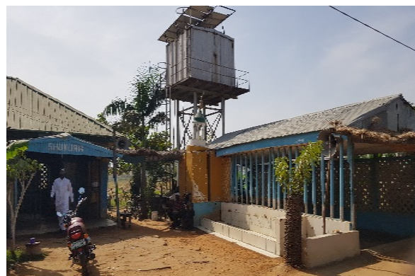
Figure 5: Public latrine along Hadejia major road for travelers
