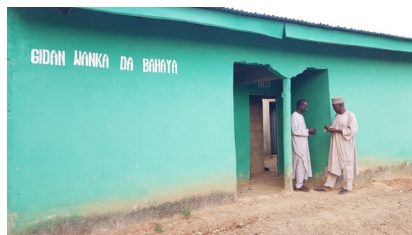
Figure 13: Public latrine managed by private sector and collecting user fees
