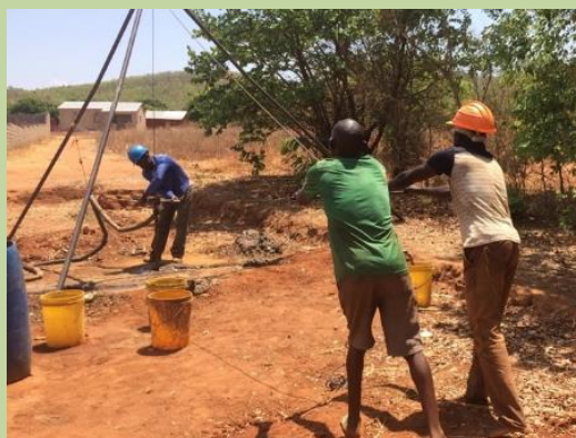
Figure: Eastern Manual Drillers drilling in Chipata peri-urban area, Tanzania (photo: Sally Sutton).
