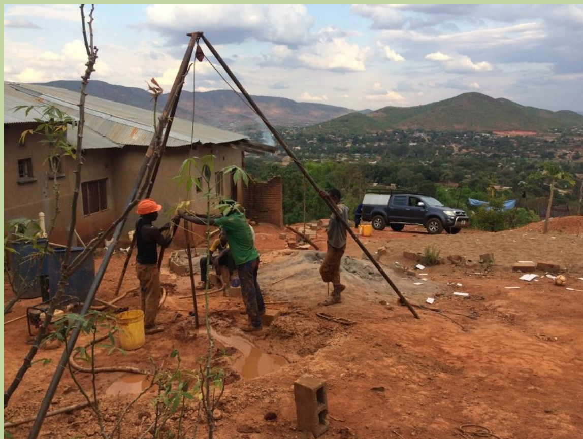
Figure (below)) Manual drilling above Chipata town (photo: Sally Sutton)
