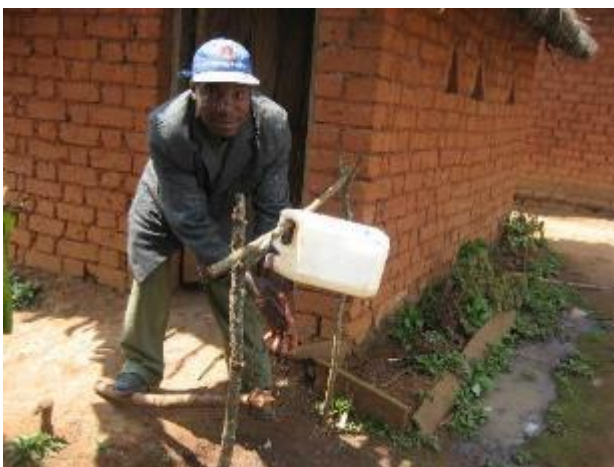
Rope of a Tippy tap may damage fast with the UV sun rays. Instead of rope, one can also use 1.5 mm galvanised wire. That last much longer than rope
