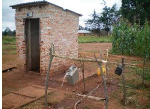
If possible install Tippy taps near latrines
