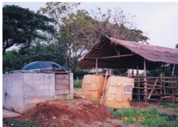
Silage making by packing chopped pasture plants in a concrete-made bunker silo (also note two large plastic bag silos next to the bunker silo, which have preventive measures against dogs) (Central region)
