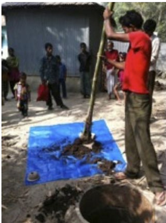
Figure 3: Manual emptying of pit latrine
