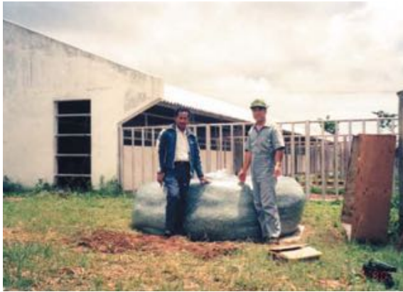
Completion of sealing work
