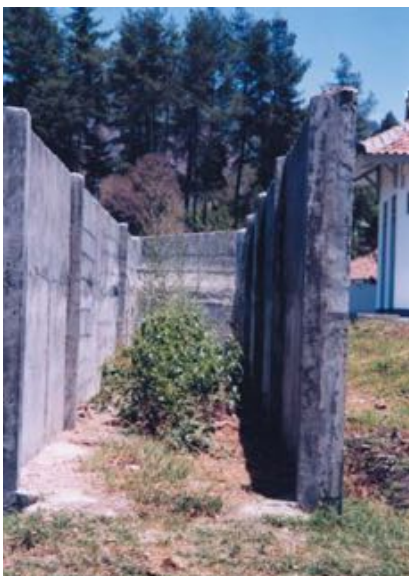
A concrete-made bunker silo (The frontage is made narrow to prevent secondary fermentation.)
