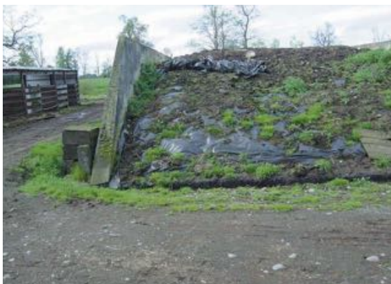
A large bunker silo in the Agricultural Experiment Station (If air tightness is maintained, storage for more than 1 year is possible.)
