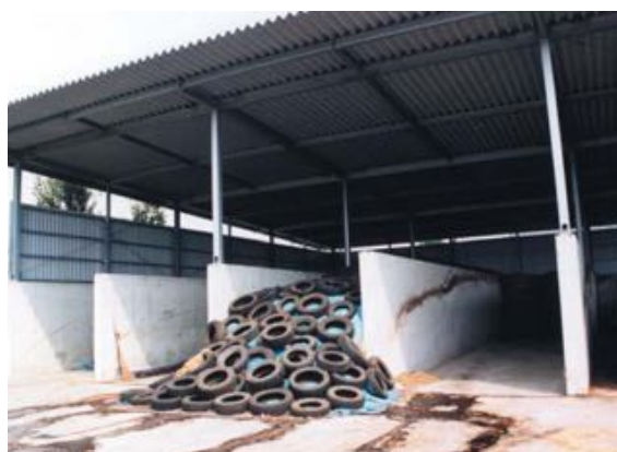
Sealing and storing in the bunker silo with a roof (the weights are old tires)
