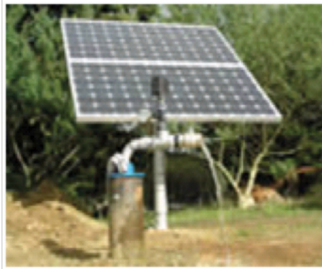
Figure 7.1 A PV Module for water pumping
