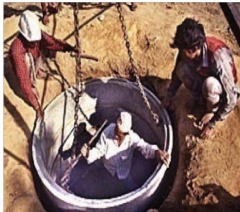
Figure 3.5 Hand Dug Well digging (Water Aid/ Picture by Caroline Penn )
