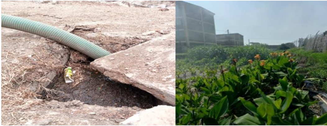
Figure 4: Septic tank (left) before and wetlands constructed (right) for sewage treatment in Shashamane. Photo credit: BBBC
