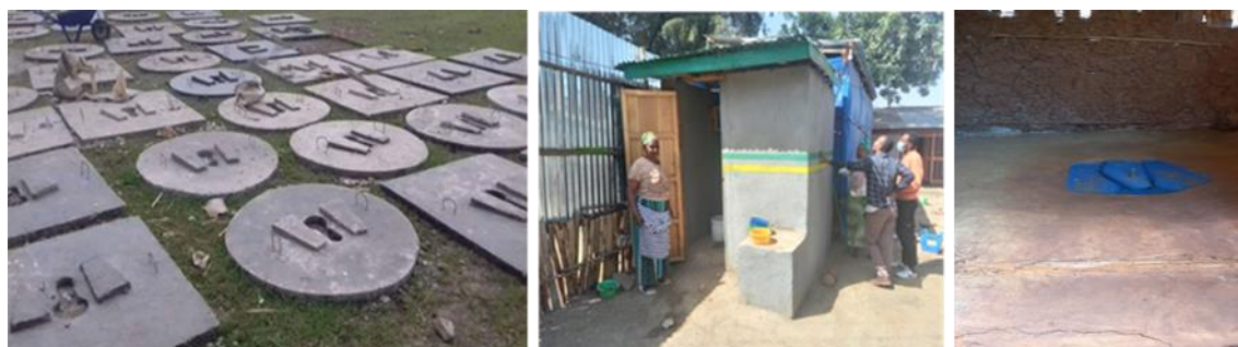
Figure 1: Slab manufacturing (left), construction of improved latrines (middle), and plastic slabs (right). Photo credit: Amref, BBBC and Plan international sub-programme offices
