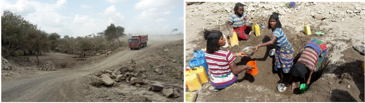
Picture 5 road diversion serving as sand-dam to support scoop holes
