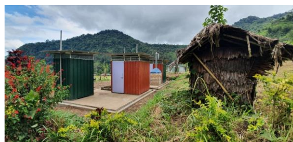
Photo 1: Climate resilient school latrines in Papua New Guinea
